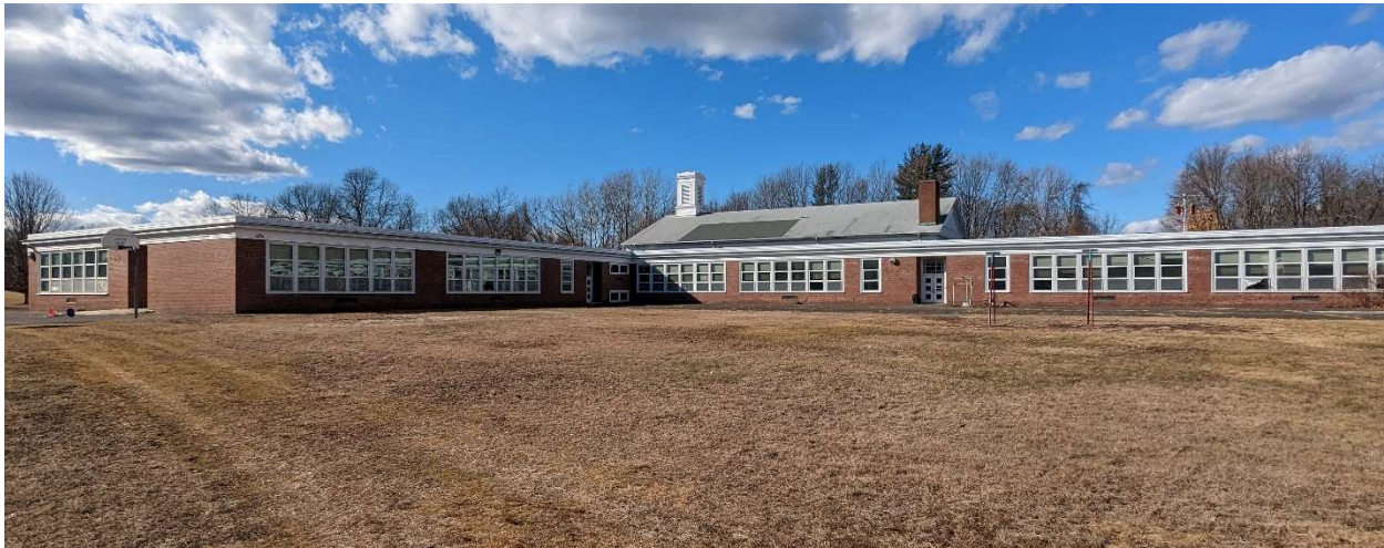
Fig. 15, 16 & 17 – view of the open field area with the remnants of the play equipment. Image of the asphalt play area.
