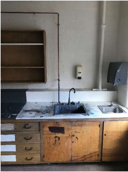
Fig.27 – Damaged Millwork
