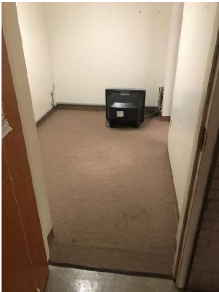
Fig.101 – Worn Carpet Floor
