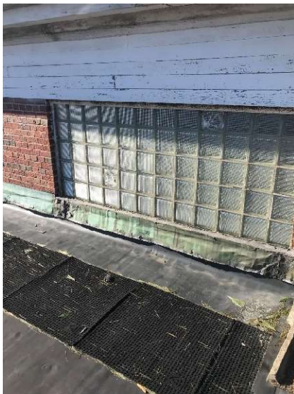
Fig.121 – Damaged flashing
