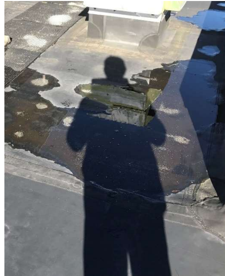
Fig.120 – ponding water
