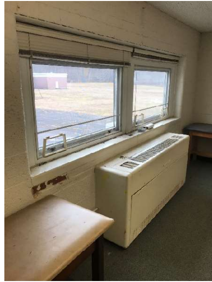
Fig.104 – Damaged CMU wall
