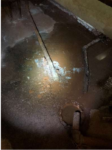
Fig. 7 – Boiler pit floor drain
