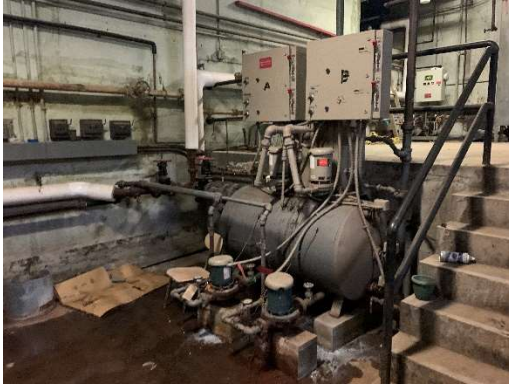
Fig 2. - Vacuum return system
