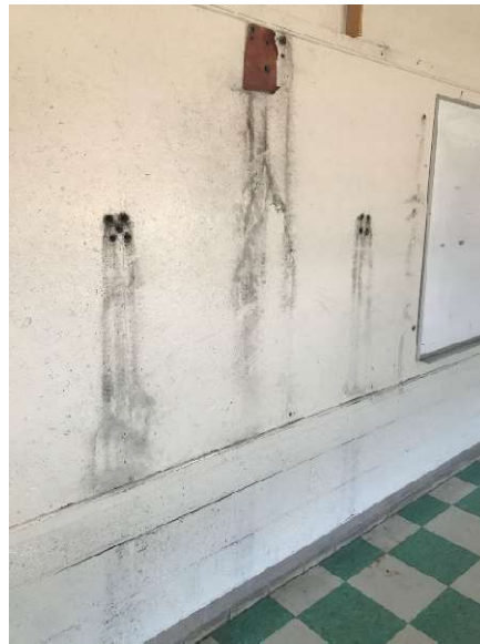
Fig.18 – Stained Wall
