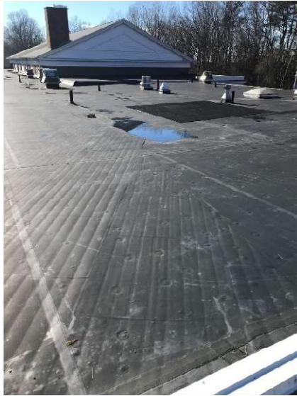
Fig.119 – Ponding water
