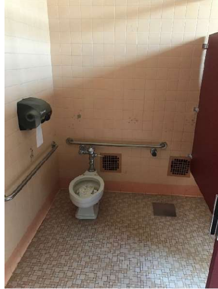
Fig.56 – Damaged ceramic wall
