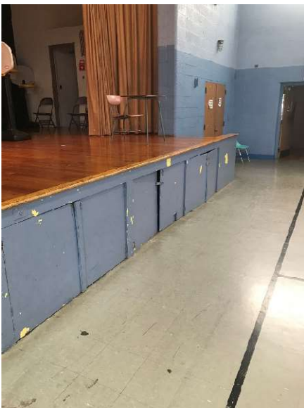
Fig.39 – Damaged Millwork
