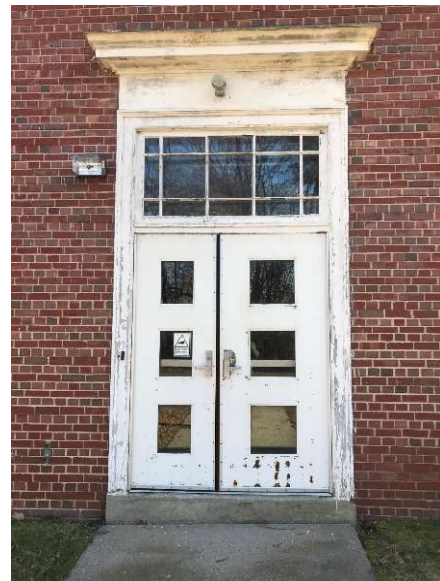
Fig.118 – Damaged door/frame/trim
