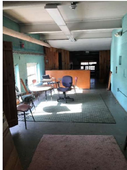
Fig.108 – Attic space view
