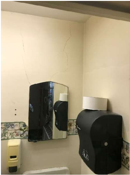
Fig.49 – Cracked wall
