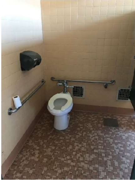
Fig.53 – Existing ADA stall
