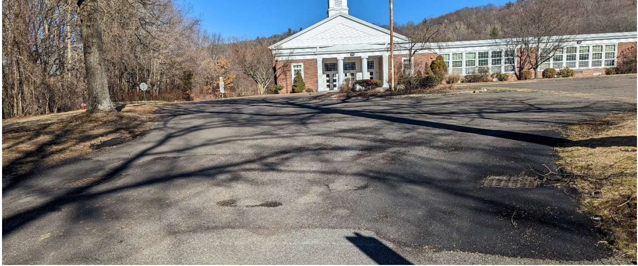
Fig. 12 – drainage structures at along the access drive
