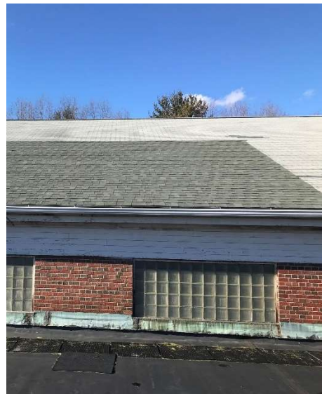
Fig.122 – Roof shingle repaired
