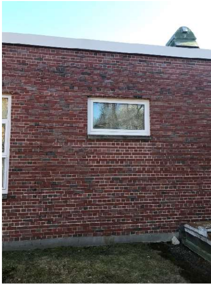
Fig.109 – Stained brick veneer wall
