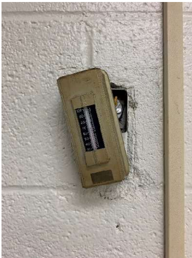
Fig. 4 – Damaged thermostat
