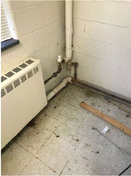
Fig.79 – Damaged vinyl tiles
